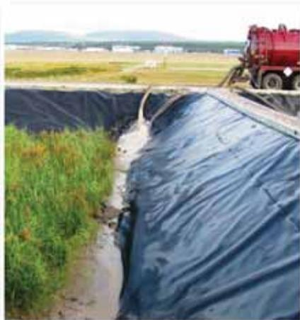
*Figure 3. Stephenville sludge treatment cells being filled.*
