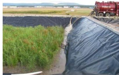
Application of sludge to sludge cell
